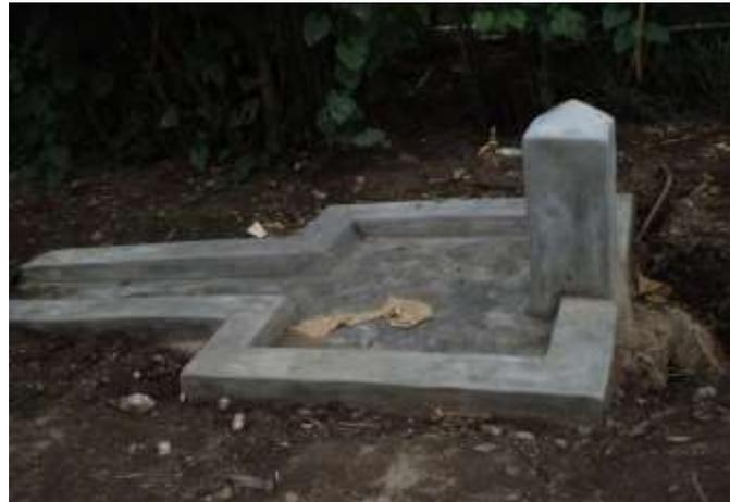
*Single faucet tapstand constructed 10m away from the tank as a fetching point*
