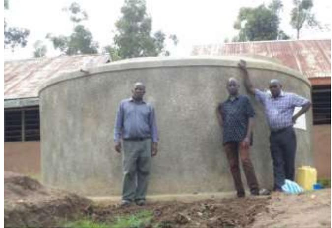
*30m<sup>3</sup> ferro-cement tank constructed and finished at Bwambara PS*
