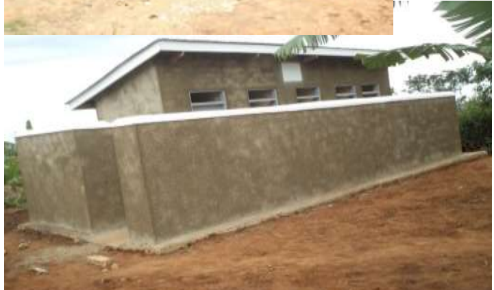
A 6 stance pit latrine for boys constructed at Bwambara SSS
