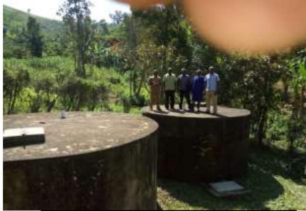
While at the Distribution/Reservoir tank
