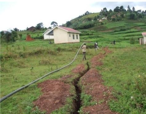
**Laying of a pipeline at Kabuga HC II before the construction of a double tanstand at this centre**
